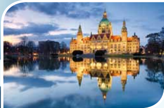
Headquarters Hanover, Germany
